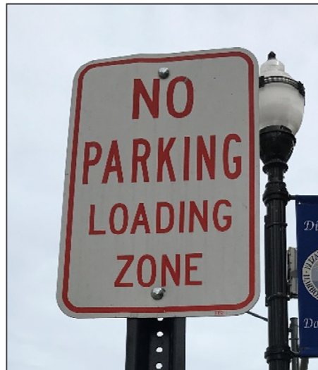
Exhibit 12: Photograph of Existing R7-6 Sign Panel
