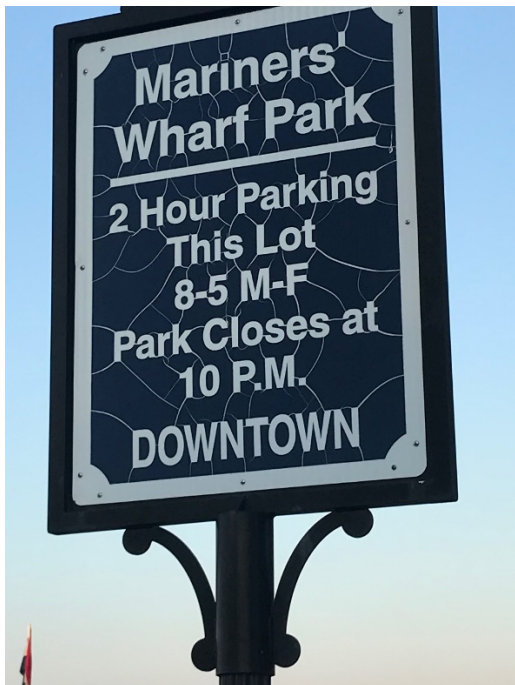
Signs that have begun to crack and show weathering
